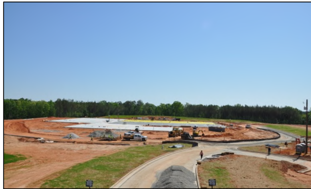
APRIL 2014 GROUND BREAKING
