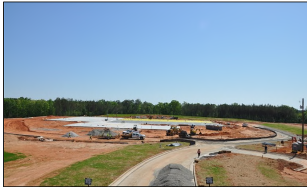
APRIL 2014 GROUND BREAKING
