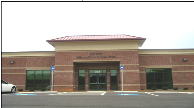
SITE VISIT NOVEMBER 2014
